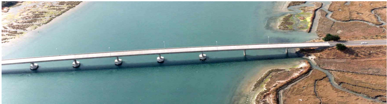
Fig. 1: Humboldt Bay Middle Channel Bridge (Courtesy of Caltrans)
